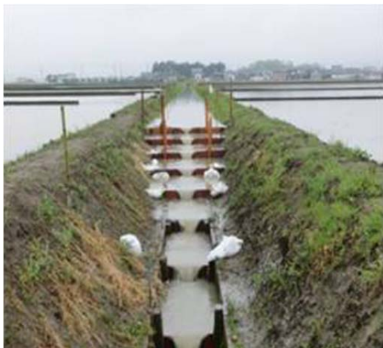
A fish ladder constructed in a drainage canal.
