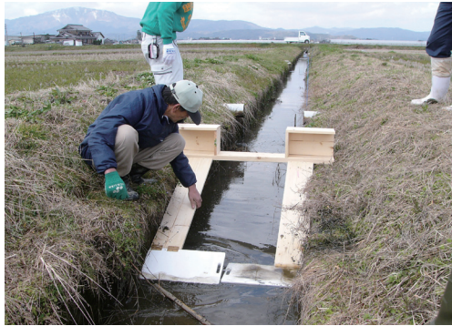
(photo 4) Kame-Kaeru slope (tortoise-frog slope) which has adjustable float with keeping slope degree as flow change
